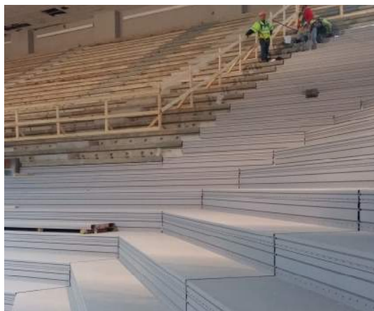
NEW LSA PAIRED WITH EXISTING PRECAST CONCRETE
