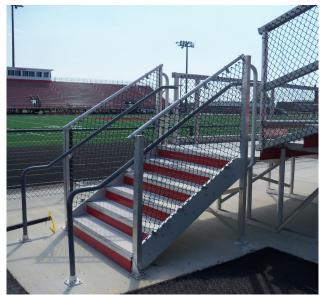
this point the cover plates for the top and front of the stair MUST BE INSTALLED per the installation drawings to cover the sharp corners to prevent injury. Install the joint cover if necessary and apply anti-skid nosing with the required number of pop rivets. Then install the grab rails and anchor to the concrete.
